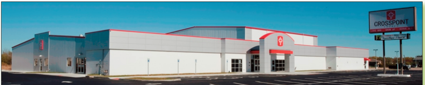
Original profile of building above. Renovated main entrance, CrossPoint Church, below. Eave height over the sanctuary portion was raised from 14' to 25' and exterior was completely redone.
